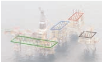
The North Sea Energy Island: 4 platforms to be retrofitted with energy infrastructure
